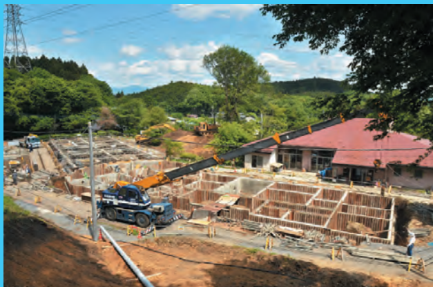
Rebuilding of Canteen
